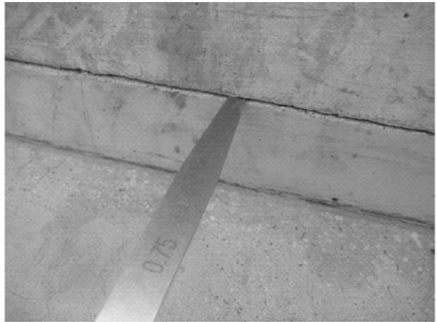
图3 沥青砂浆离缝、缺损
